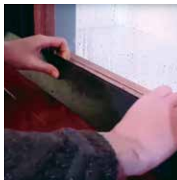
The cover profile is easily clicked open.
